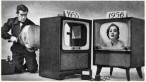
SERVICE TECHNICIAN installs a new "100 Series" G-E Aluminized Tube in the 'S3 set—tests receiving tubes, replaces weak ones with new General Electric Service-Designed tubes. Now same light netter proves the 3-year-old set outperforms the 1956 television with its non-aluminized picture tube.
